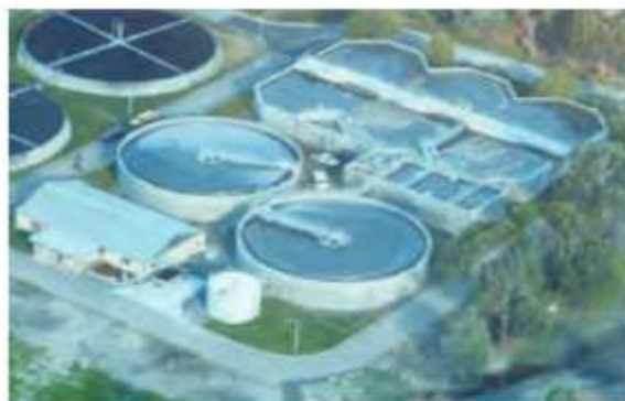
Figure 8.7 An aerial view of a sewage plant
